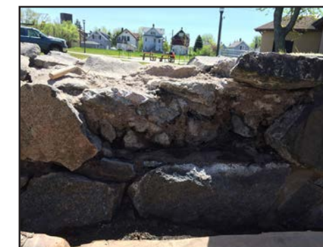
Removing Loose Rocks
