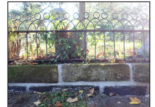
Stone Wall - After
