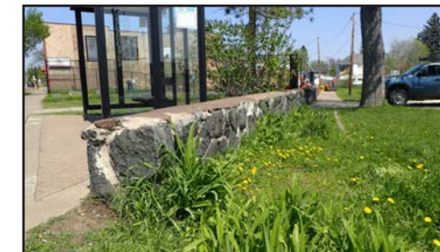
Rock Wall - Before
