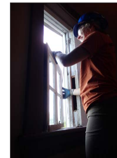
Water Tower - During
