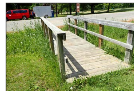
Pedestrian Bridge - Before
