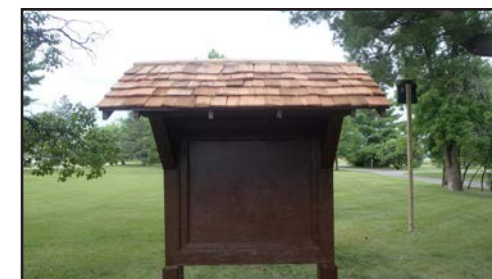
Supervisor’s Office Kiosk - After
