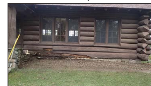
Pavilion Ramp - After
