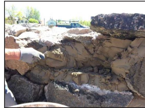
Mortar for Placement
