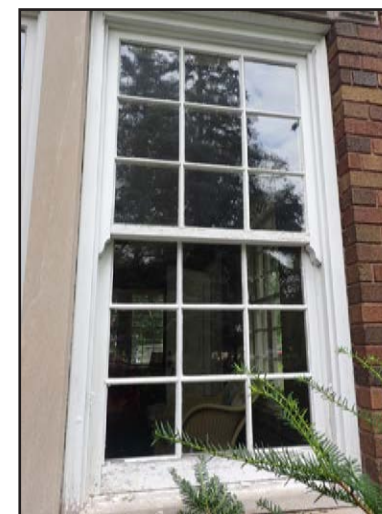
Main House - Before
