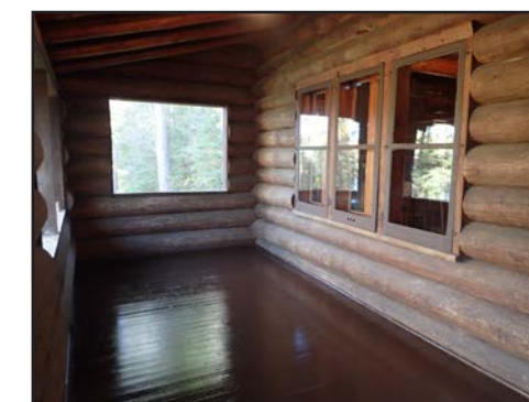
Porch Floor - After
