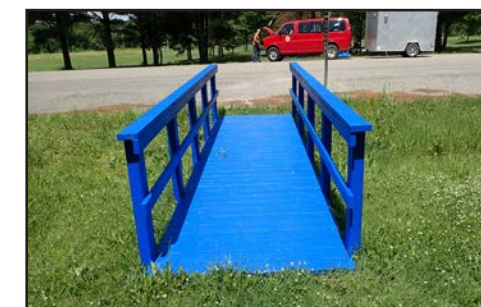
Pedestrian Bridge - After
