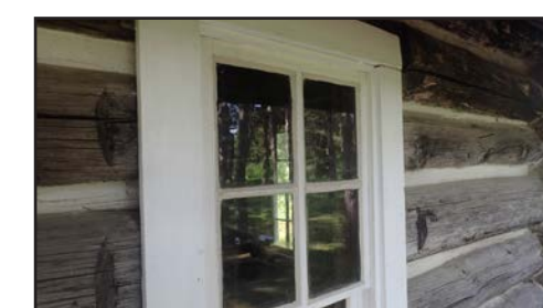
Cut Foot Sioux Ranger Station - After
