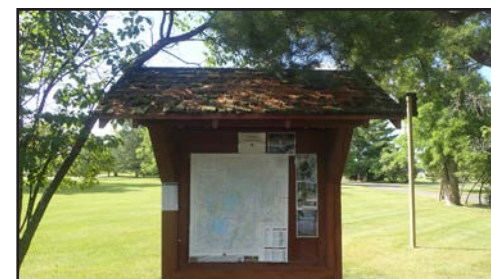
Supervisor’s Office Kiosk - Before
