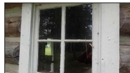
Cut Foot Sioux Ranger Station - Before
