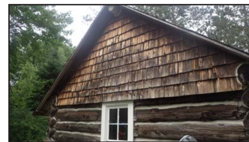
Cut Foot Sioux Ranger Station - Before
