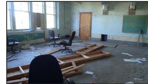
Second Floor Room - Before
