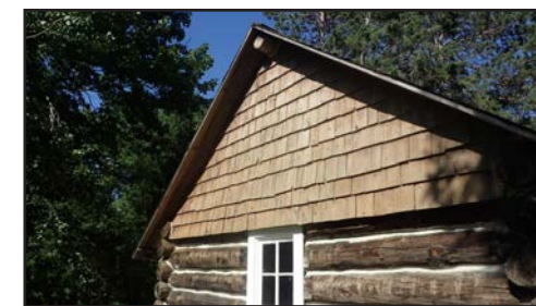
Cut Foot Sioux Ranger Station - After
