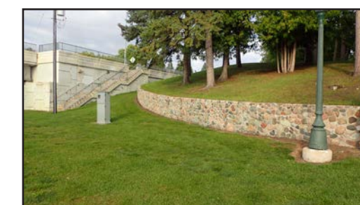
Stone Wall - After
