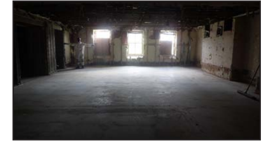
First Floor - After
