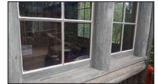
Point Cabin - After
