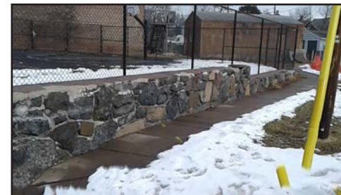
Site Visit - Before
