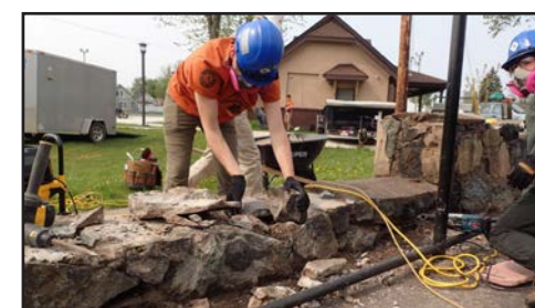
Removing Loose Rocks
