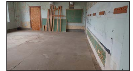
Second Floor Room - After
