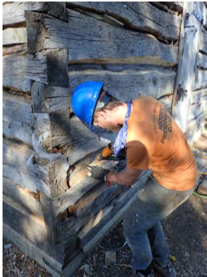
Securing Metal Lath
