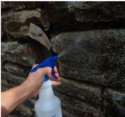
Cleaning the Stones
