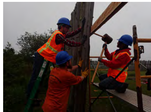
Securing Dowels
