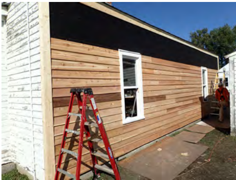
New Siding and Window Frames
