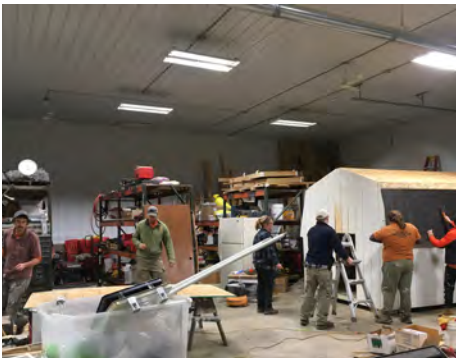
Building a Shed
