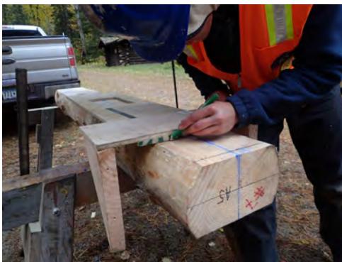
Measuring Dovetails
