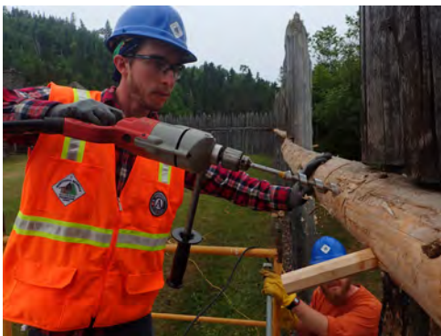
Drilling Holes for Dowels
