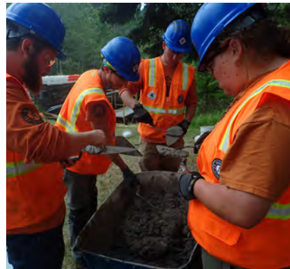
Mixing Mortar "Mud"
