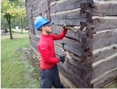
Removing Old Daubing
