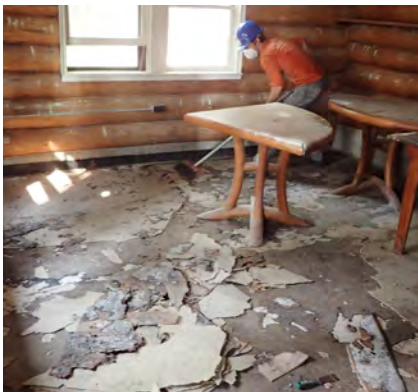
Removing District Office Floor
