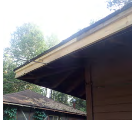
Fascia Board- After
