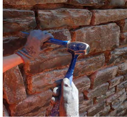
Removing Old Mortar
