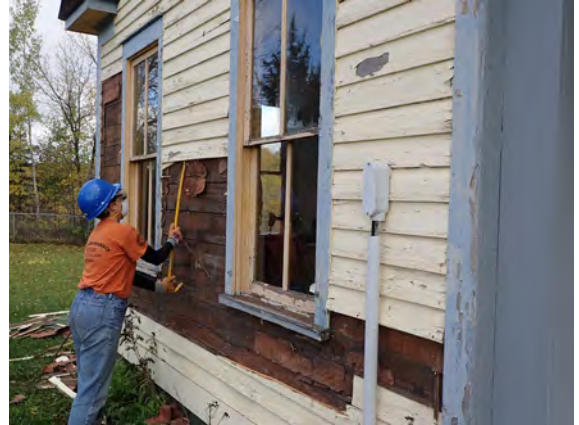
Removing Siding
