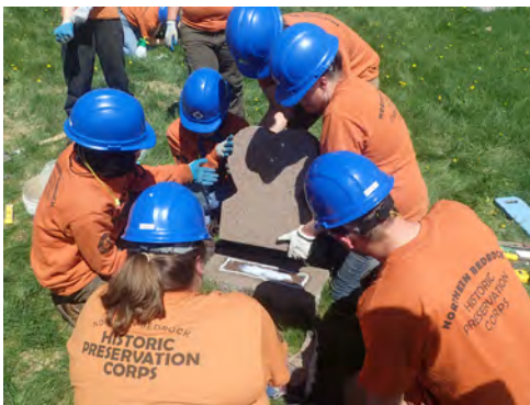
Setting Compound and Epoxy
