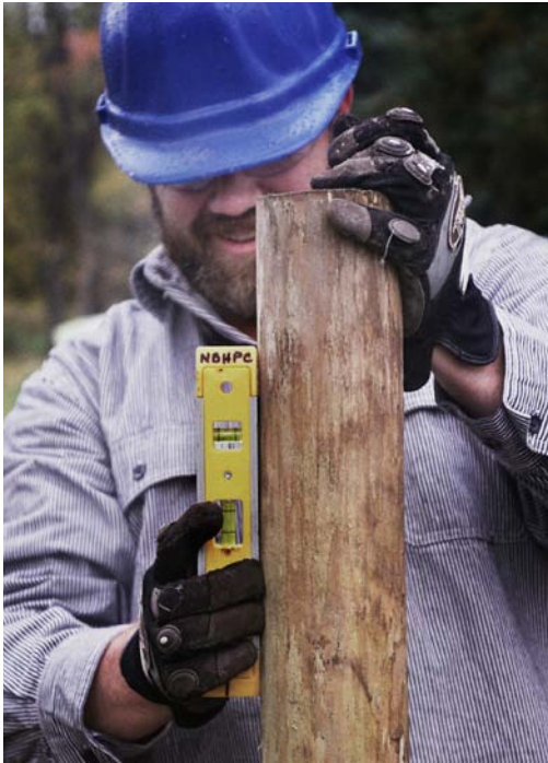
Operations Director, Pete Bonk, checks for verticality before securing a new fence post at Hay Lake School.
