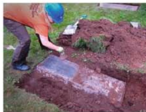
Carlton Hillside Cemetery (Carlton, MN): A double-length stone being restored by a crew member removing grass overgrowth, levels the marker and cleans the lettering.
