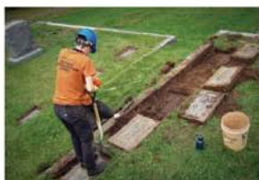
Carlton Hillside Cemetery (Carlton, MN): Crew members use guidelines to ensure markers are placed straight.
