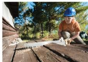
Prairie Portage - Superior National Forest: Crew member Jeannie Collins shortens logs not under the roof's eaves to prevent rot.
