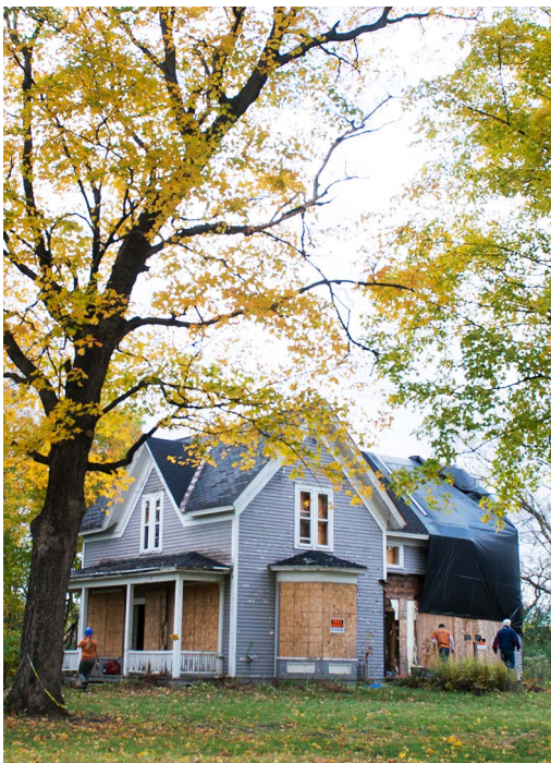
The Boutwell House in Stillwater, MN was partially demolished in January 2015.
