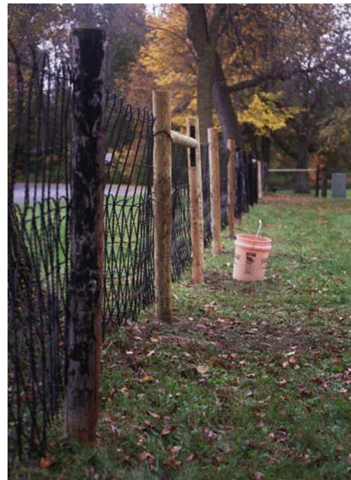
Replacing the rotted fence posts outside the Hay Lake School will ensure the fence stands for decades to come.
