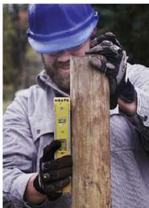
Hay Lake School & Erickson Log Cabin: Operations Director, Pete Bonk, checks for straightness as the fence post is installed.
