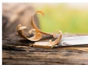
Prairie Portage - Superior National Forest: A replacement plug is chiseled down readying it for the epoxy process.
