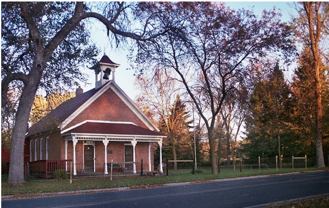
Hay Lake School in Scandia, MN after repairs to the fence were completed by the Northern Bedrock crew. Photo by Ashley Brey.
