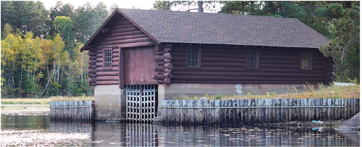
USFS Lac La Croix Boathouse, built by the Civilian Conservation Corps in 1937. The exterior wall facing the lake was the only wall not refinished during the crew's visit, due to safety concerns.
