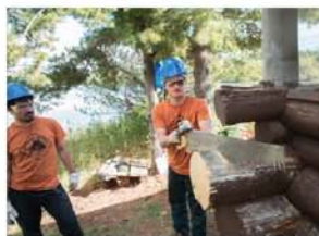
Prairie Portage - Superior National Forest: Crew leader Josh Preston looks on as crew member Ryan Larson shortens water-damaged logs.
