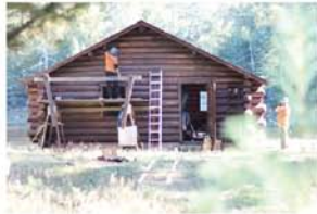
Lac La Croix - Superior National Forest -- Crew on scaffolding and around cabin applying a protective oil-based stain.
