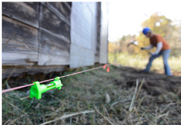
Creating a slope away from the foundation of the barn.
