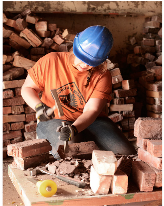
Lexi using rock hammer and chisel to remove mortar.
