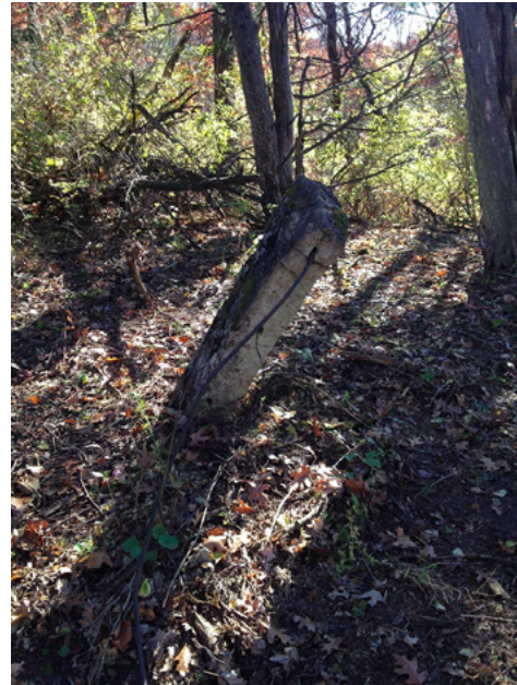
A sunken crooked stone fence post surrounding the Sherwood plot at Oakwood (Sherwood) Cemetery in Rushford Village, MN.
