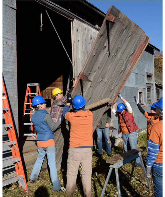
Lowering the doors to sawhorses to begin restoration.
