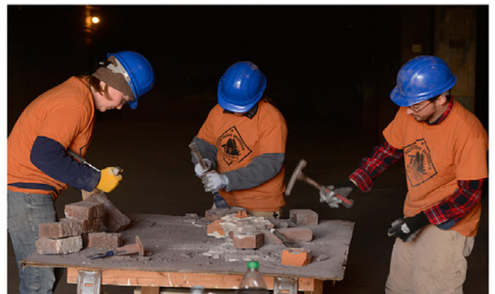
Anne, Meghan and Zach removing mortar to ready bricks for reuse.
