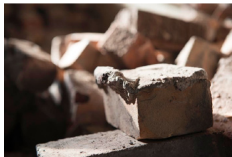
A brick covered with dried mortar requires cleaning before it can be reused with fresh mortar. The crew worked for two days and cleaned around 1,750 bricks. A huge help to the masons working on the restoration of the parapet walls.
