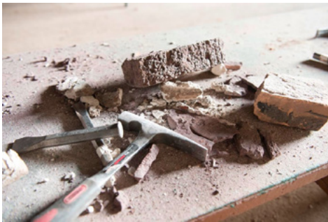
Tools used at the Duluth Armory to clean dried mortar from bricks include a brick hammer and chisels.
