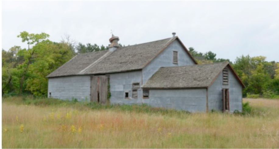
The northeast side of the McDougall Barn, August 2014.
