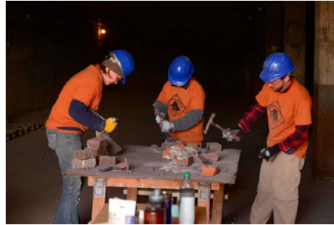
Crew leader Anne Ketz working with crew members Meghan Weber and Zach Small cleaning bricks at the Duluth Armory.
