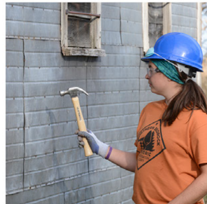
Meghan securing the metal siding.
