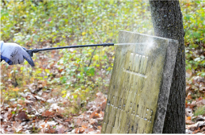
Crew uses water and D2 solution to clean stone monuments.
