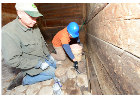
Technical specialist Paul Ormseth, architect, teaching crew member Zach Small how to install mortar around
