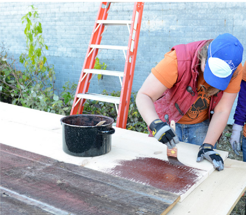
Using paint made of traditional ingredients, Lexi paints the replacement boards.
