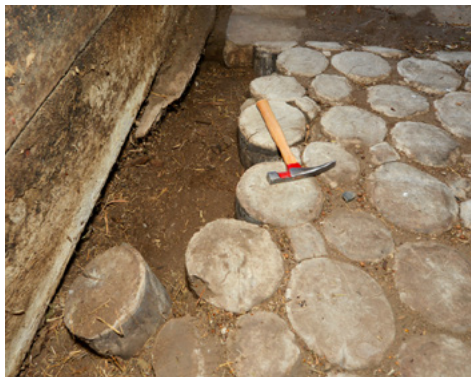
Horse stall floor, west end of McDougall Barn, prior to repairs.
