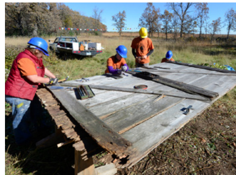
Crew members Lexi Kosik and Jennifer Sustar removing deteriorated boards from the east door of the McDougall barn under the direction of timber framer Adam Valesano.
