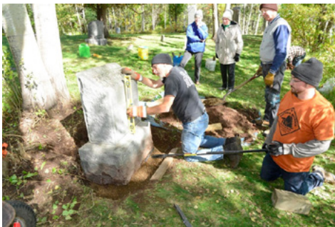
Crew member Zach Small working with workshop participants in resetting a sunken stone at Scandia Cemetery.
