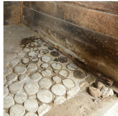
Repairing the floor with lime mortar.
