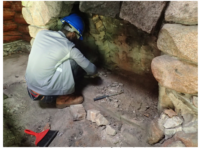
Repair work on the firebox begins
