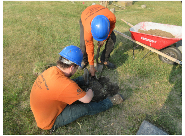
Cemetery restoration in progress
