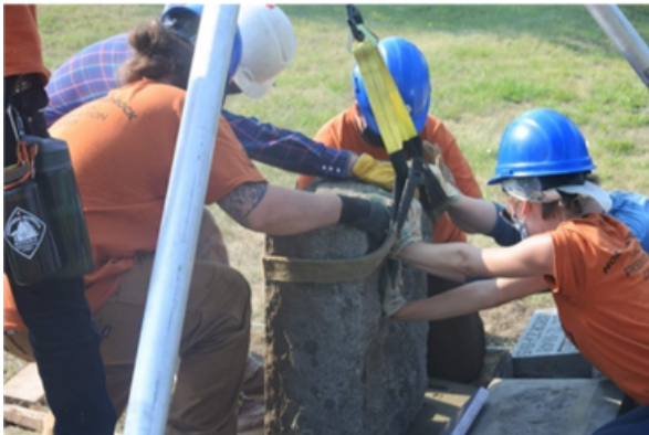
Corpsmembers learn how to safely and accurately lift and reset stone monuments.
