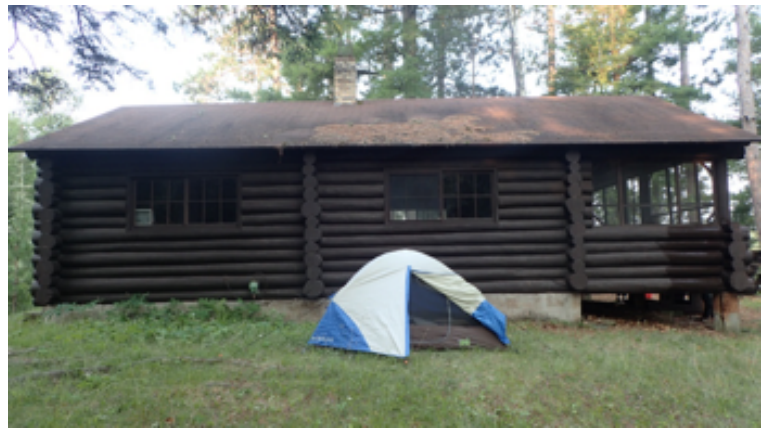
Before any work undertaken on the Guard Station at Sawbill.
