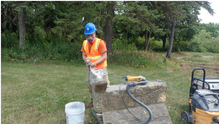
The salvaged masonry table bases needed cleaning prior to reinstallation.
