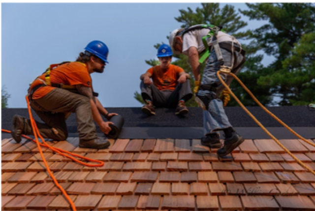
Installation of cedar shakes followed procedures outlined by the Cedar Bureau.
