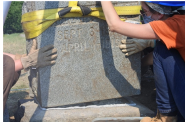
Resetting headstones on newly leveled bases. Specific monument setting putty and lead wedges are used.
