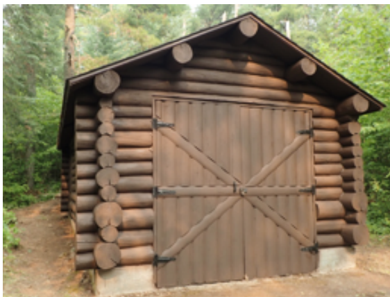
After work was complete.
