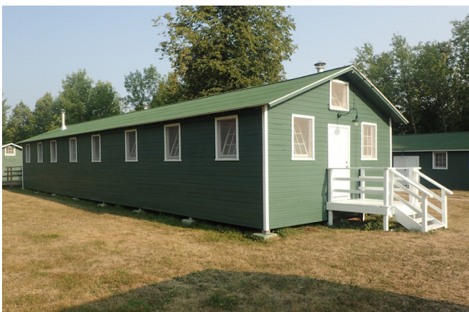
Building #5 after the exterior was refinished.
