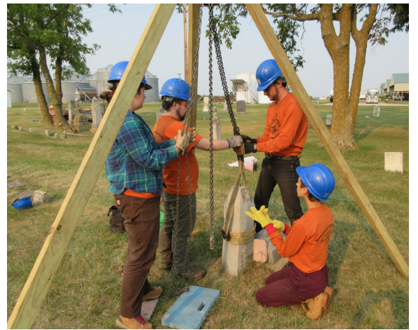
A headstone is reset using a tripod and block and tackle.
