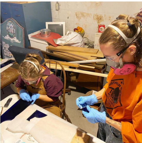
Much of the original stained glass needed to be reassembled with epoxy. Care was taken to select an epoxy with the same light refraction properties as glass.
