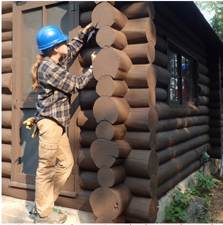
A Corpsmember paints the log ends on the Guard Station.
