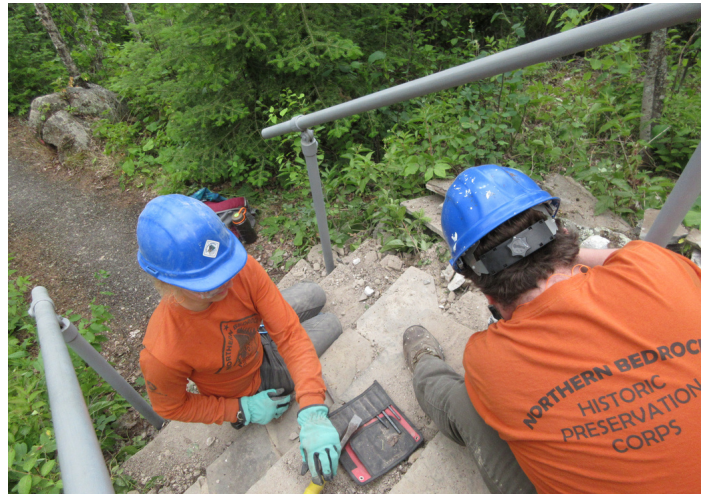
Corpsmembers begin work on restoring the masonry stairs.
