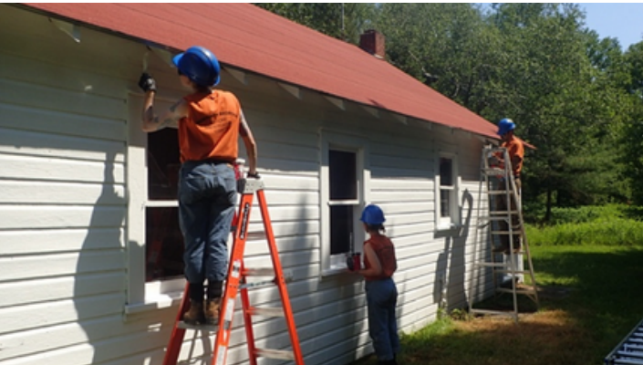
Repainting the exterior
