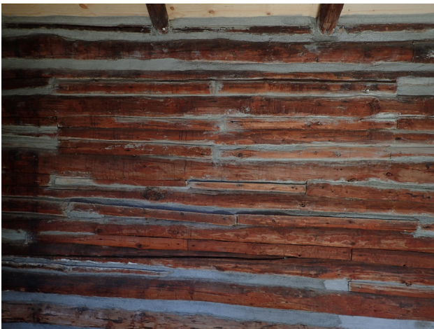
Interior wall after rechinking.
