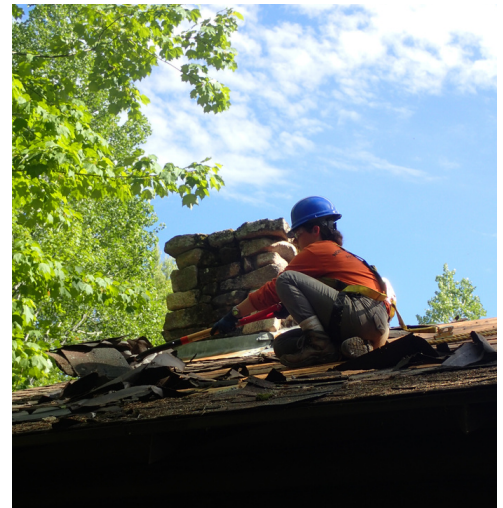
New flashing installed around original chimney
