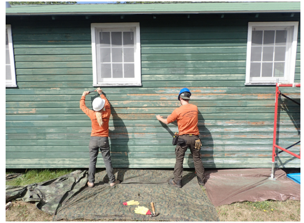
Members scrape the south elevation of Building #5, Barracks.
