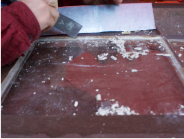
Lost Lake - Corpsmember working to remove the old finish and glazing putty.
