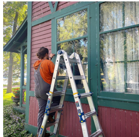
Installing a new storm window.
