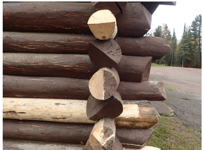
Picture showing the half log replacement.
