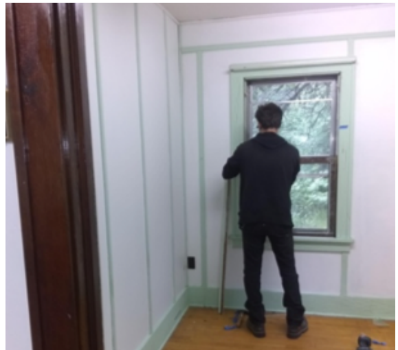
Re-installing the restored window sashes
