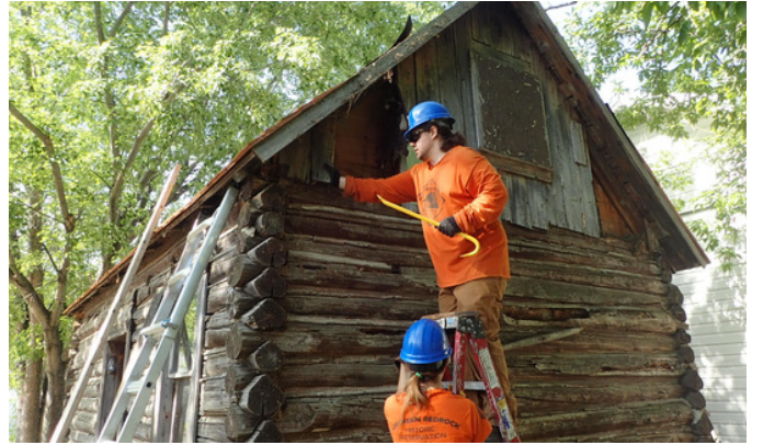
Corpsmembers removed unsympathetic siding on the north gable.
