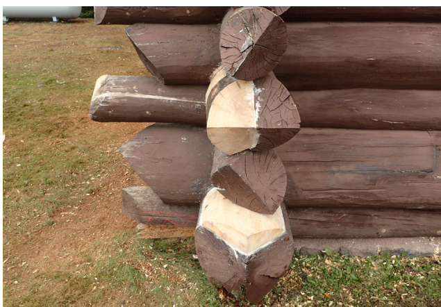
Log ends displaying 'Dutchmen' replacing half of log ends.
