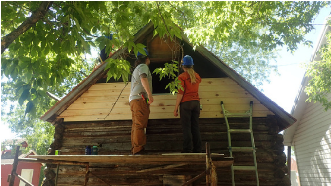
The replacement siding was milled locally to match the original found on the south gable.
