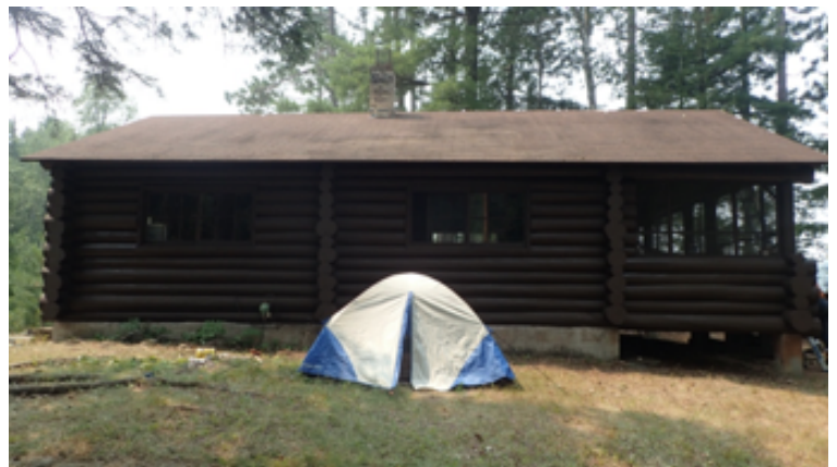
After exterior refinishing and roof sweeping.
