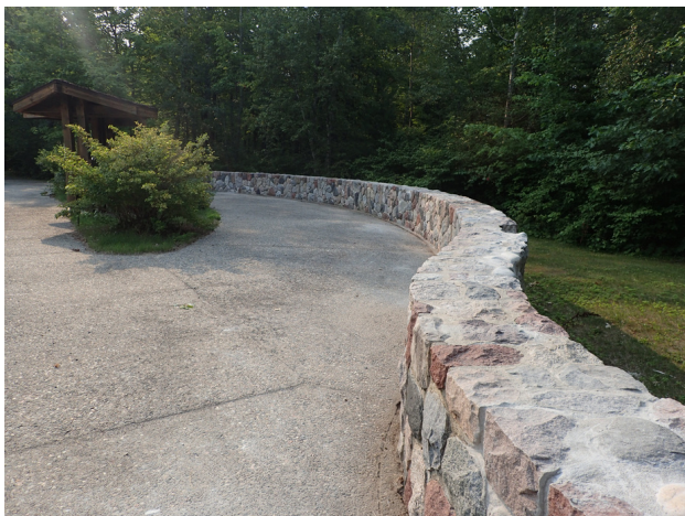
The same portion of wall after restoration work.
