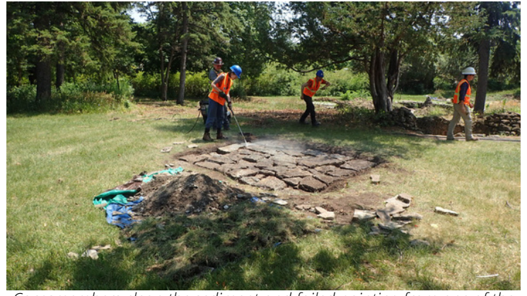
Corpsmembers clean the sediment and failed pointing from one of the original picnic table pads.
