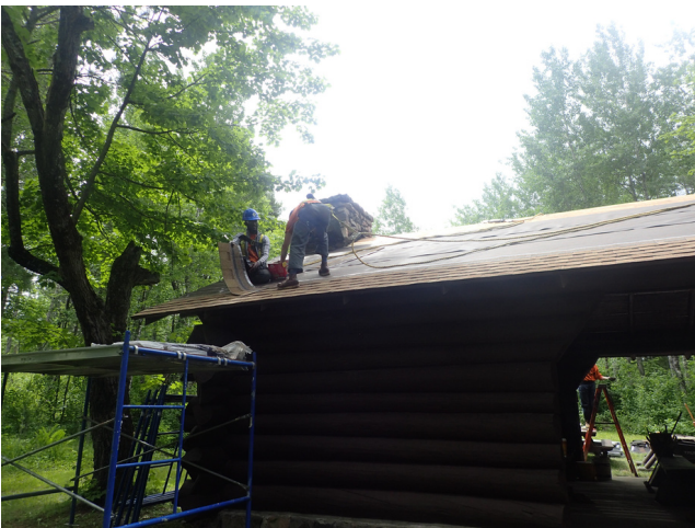
New asphalt shingles installed
