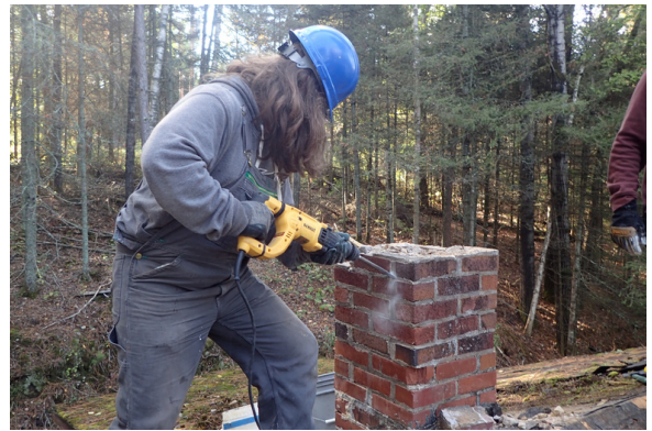
A crew member deconstructing the chimney.
