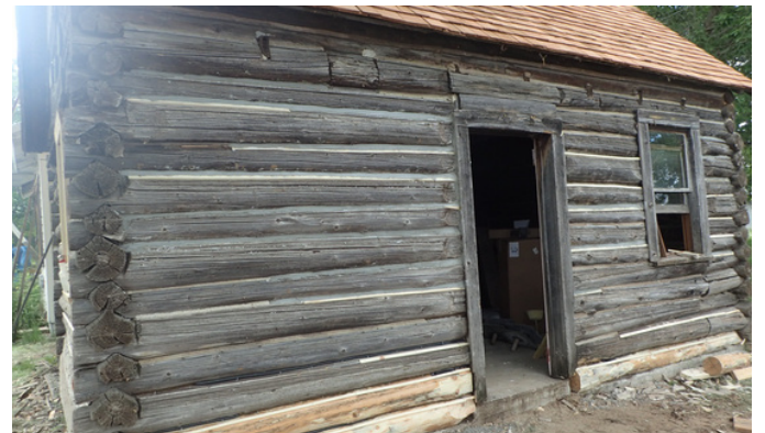
The bottom logs on the east wall were replaced
