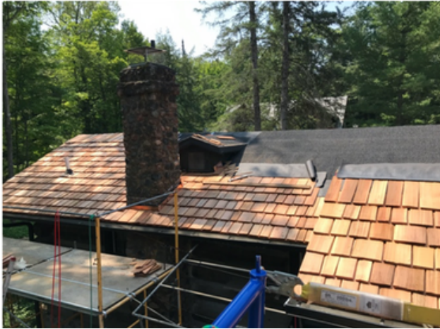
A view of the project roof as seen from the scaffolding.
