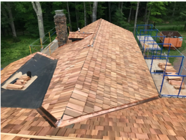
A nearly completed roof.
