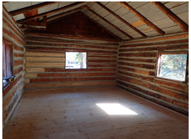
Finished cabin floor.
