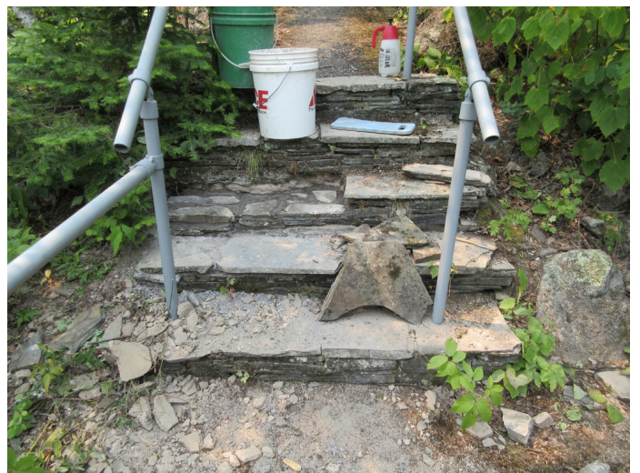
During restoration work.
