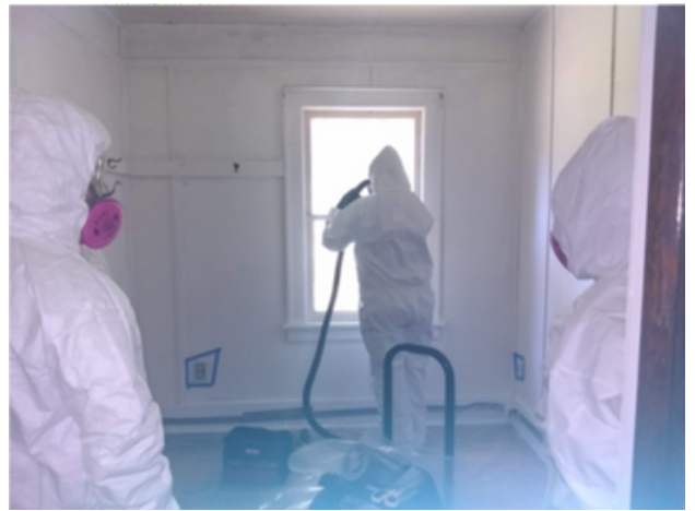
Working in PPE, Corpsmembers removed sashes
