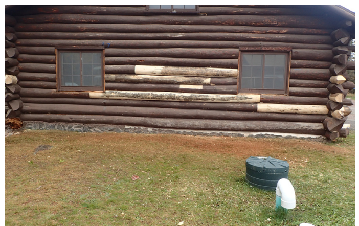
The finished log replacements.
