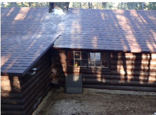
East elevation of the finished roof
