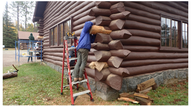
Log end being replaced.
