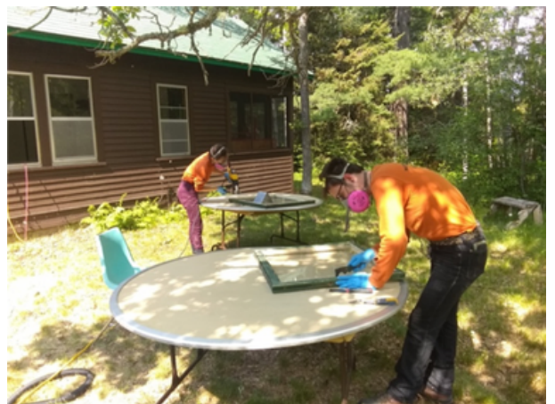
Window sash restoration
