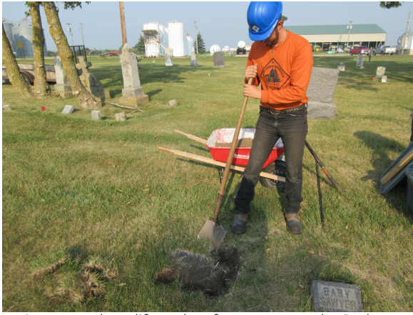
Corpsmembers lift sunken foot-stones at the Perham Municipal cemetery during restoration work.
