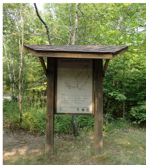
The re-roofed kiosk.
