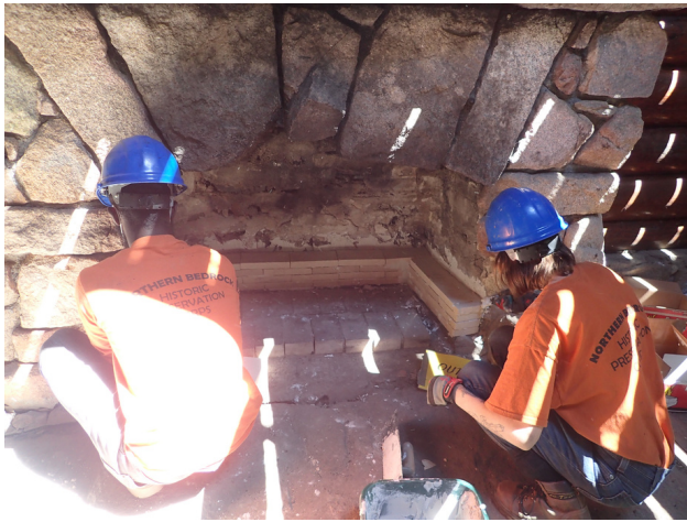
Repair work continues on the fire box
