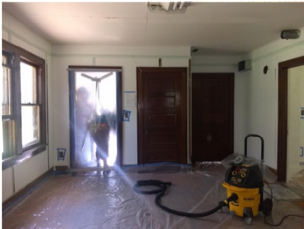
Work area was prepped
