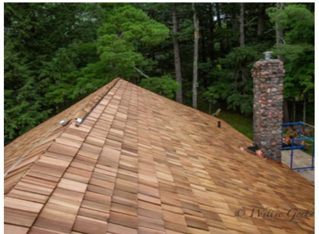
A nearly completed roof.
