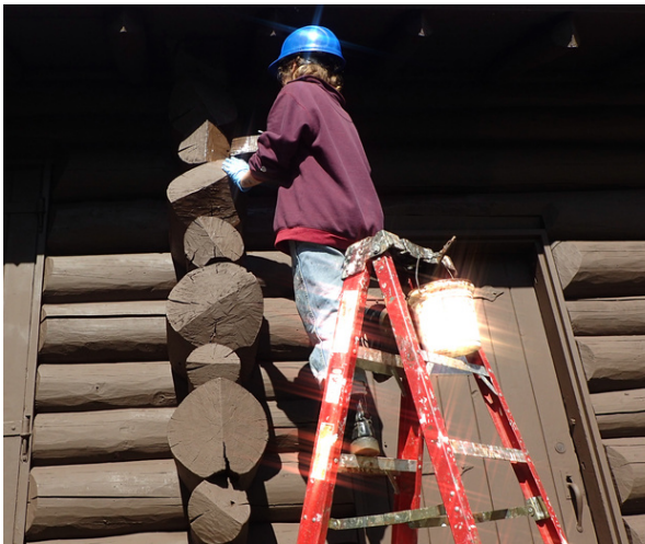
Corpsmember staining log ends on the boathouse.
