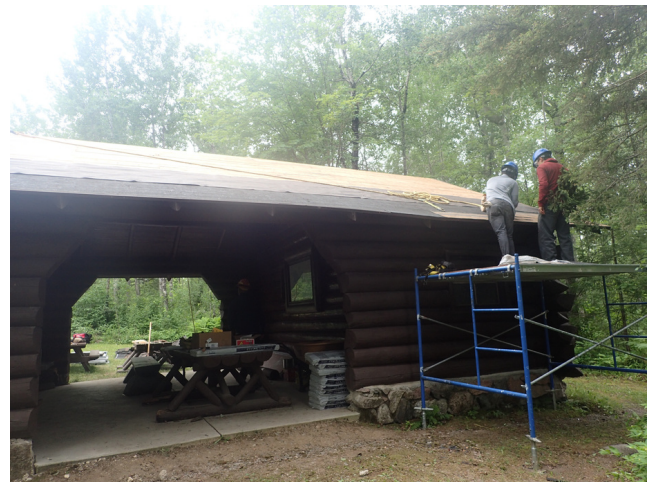
Eave access was achieved off of scaffolding
