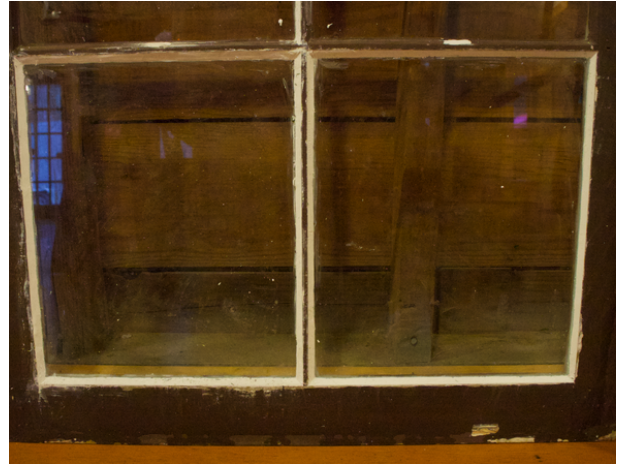
Lost Lake - Window with new glaze and prepped for finish.
