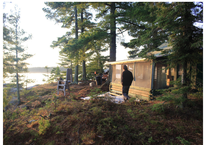
The east elevation of Fujita mid-restoration at sunrise.
