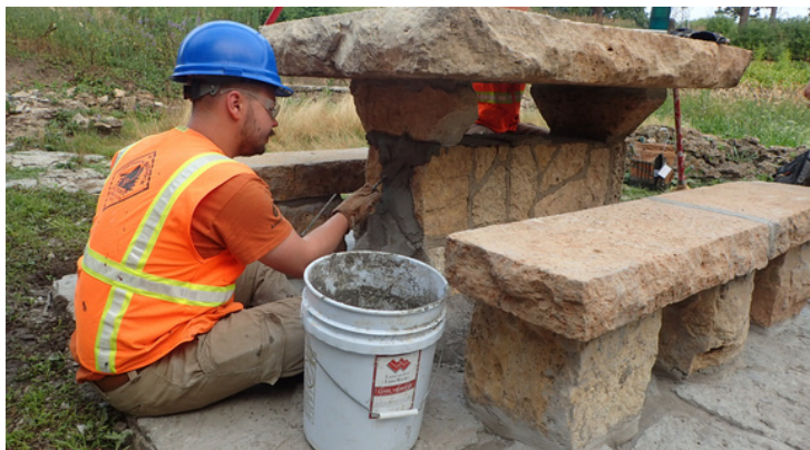
Repointing portions of the picnic table base
