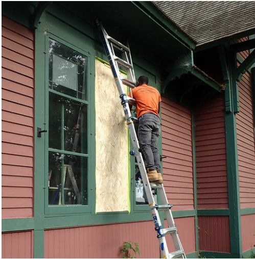
A Corpsmember temporarily boards up a window opening during restoration.
