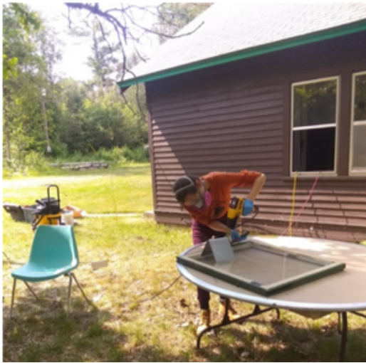
Window restoration work continued where the previous Hitch left off.
