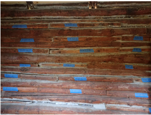
Chinking labeled prior to removal and subsequent replacement.
