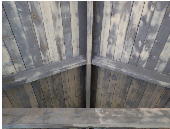
Interior underside of picnic pavilion prior to staining.
