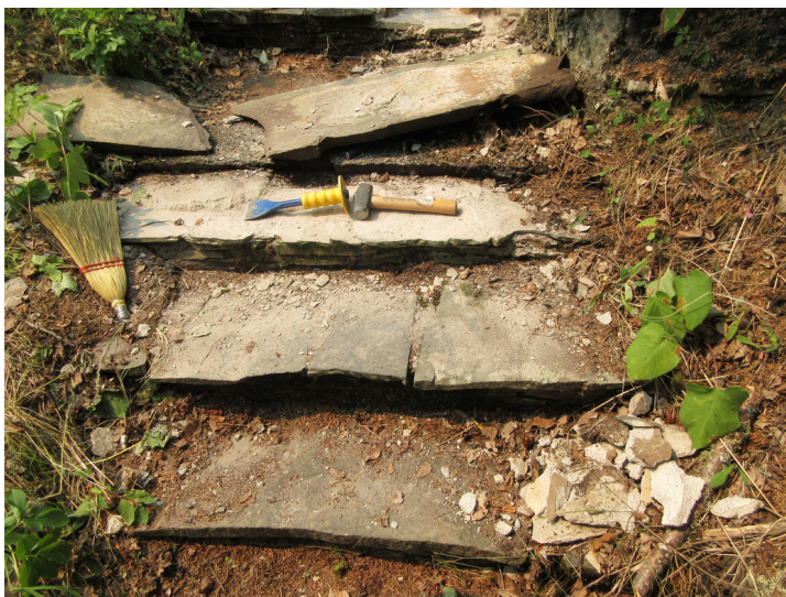
Stairs during restoration.
