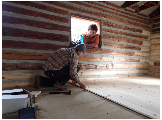
Tongue and groove flooring going in over the subfloor.
