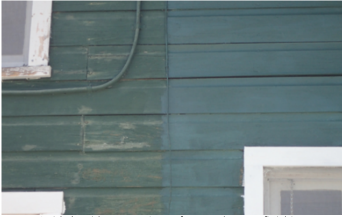
A side by side comparison of pre and post refinishing.
