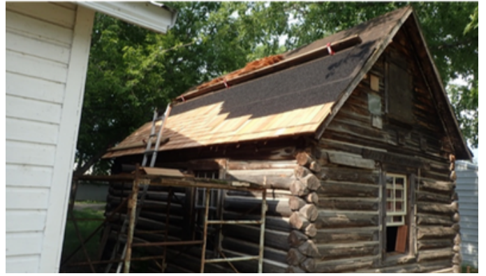
The first courses of cedar shingles installed.
