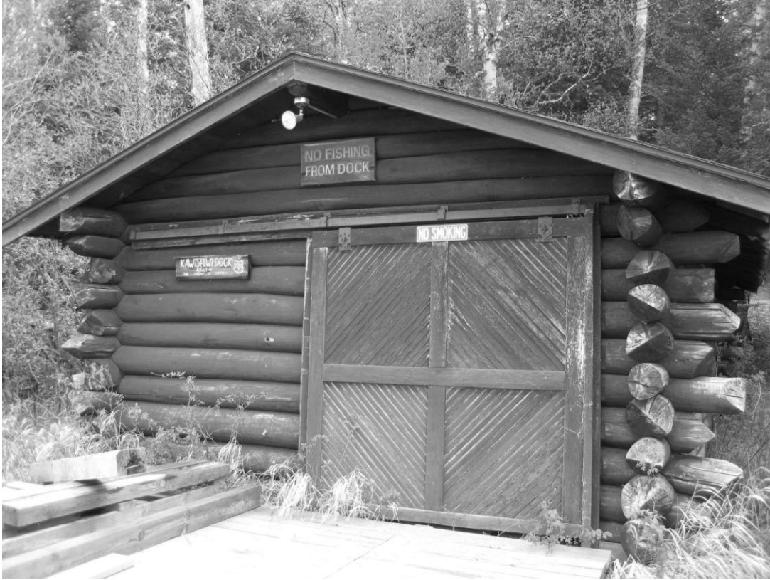
7 of 18. Boat House (FS Bldg. #31107); Contributing. Western elevation. Lake County, MN.
