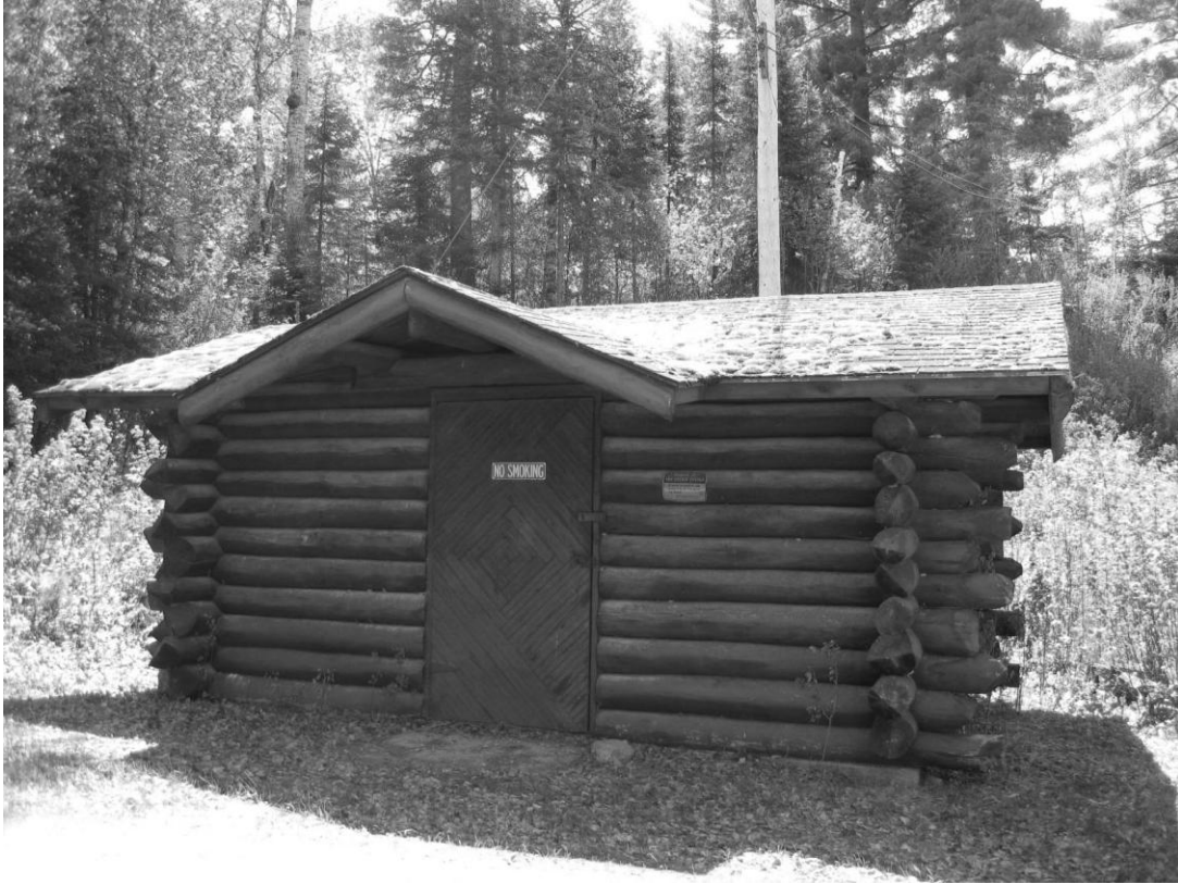
11 of 18. Oil House (FS Bldg. #31111); Contributing. Northern elevation. Lake County, MN.
