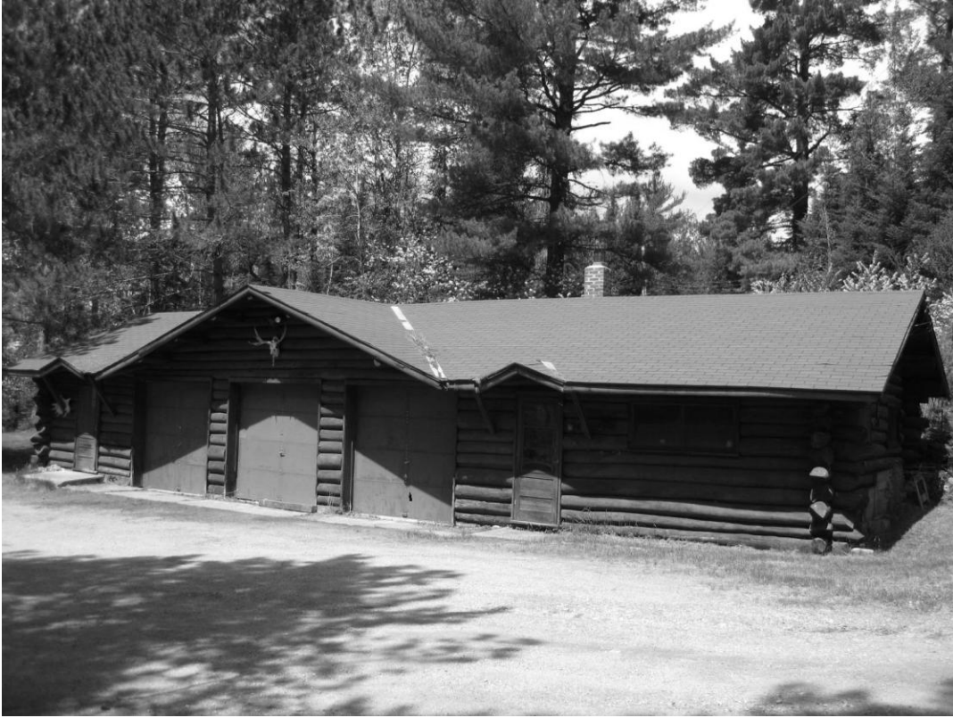
9 of 18. Warehouse (FS Bldg. #31106); Contributing. Southeast elevation. Lake County, MN.
