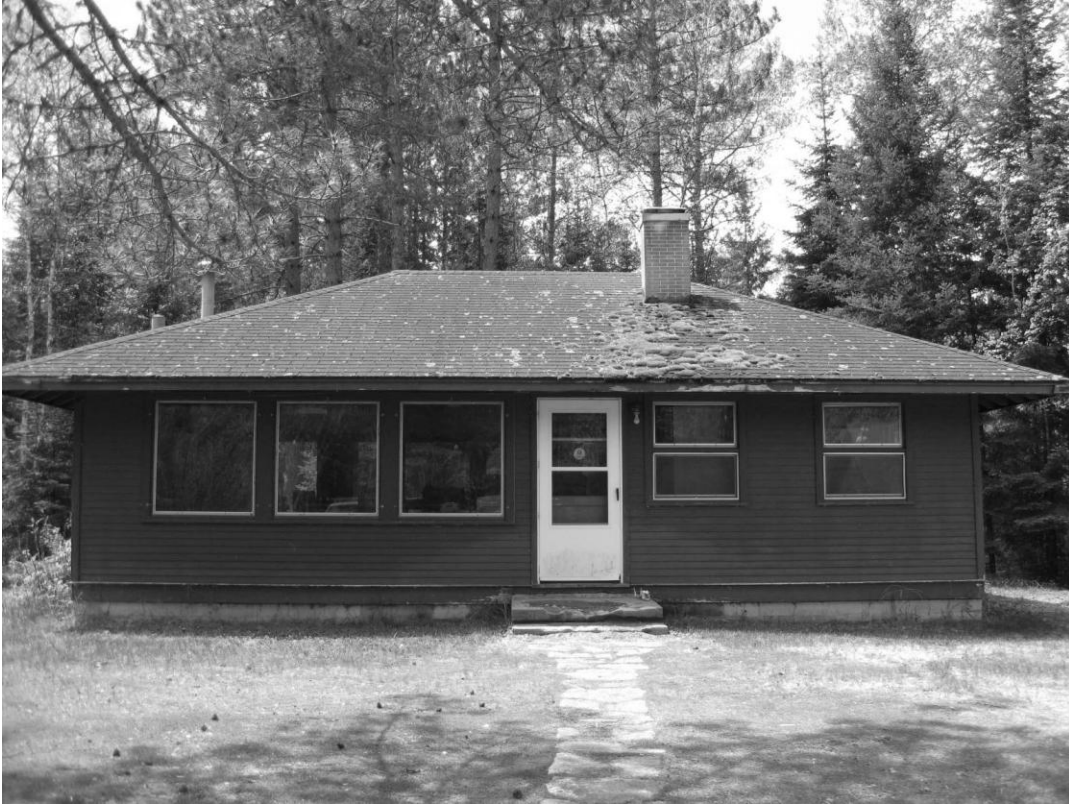
17 of 18. Laboratory (FS Bldg. #31104); Contributing. Eastern elevation. Lake County, MN.
