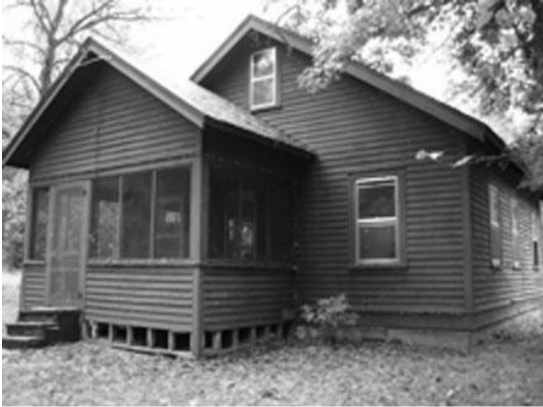
3 of 18. LSFES Office (FS Bldg. #31108); Contributing. Western elevation. Lake County, MN.
