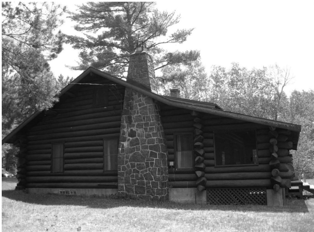
2 of 18. Ranger Dwelling (FS Bldg. #31101); Contributing. Southern elevation. Lake County, MN.
