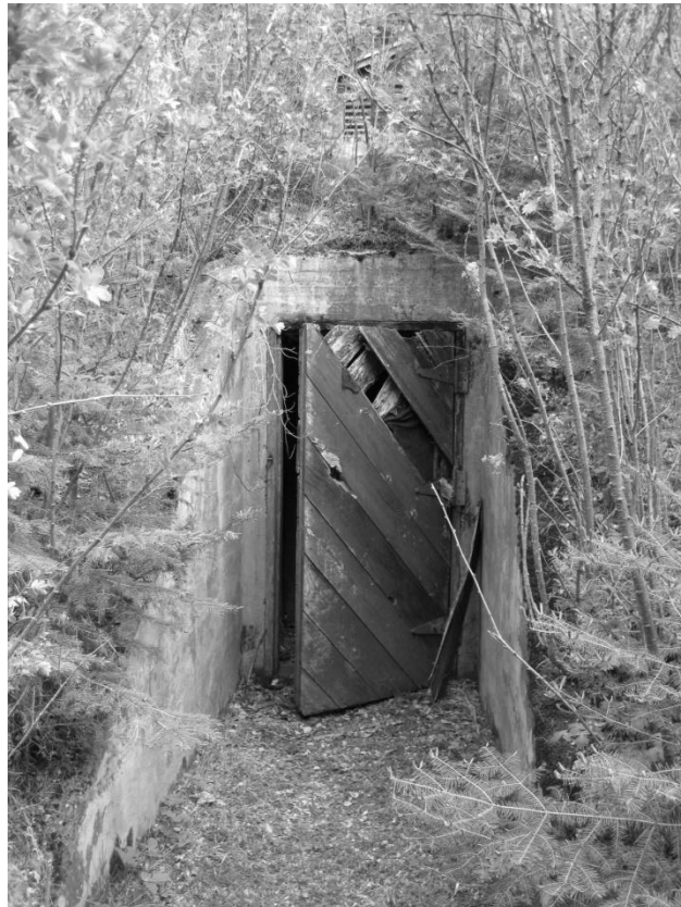
6 of 18. Cellar (FS Bldg. #31103); Contributing. Western elevation. Lake County, MN.
