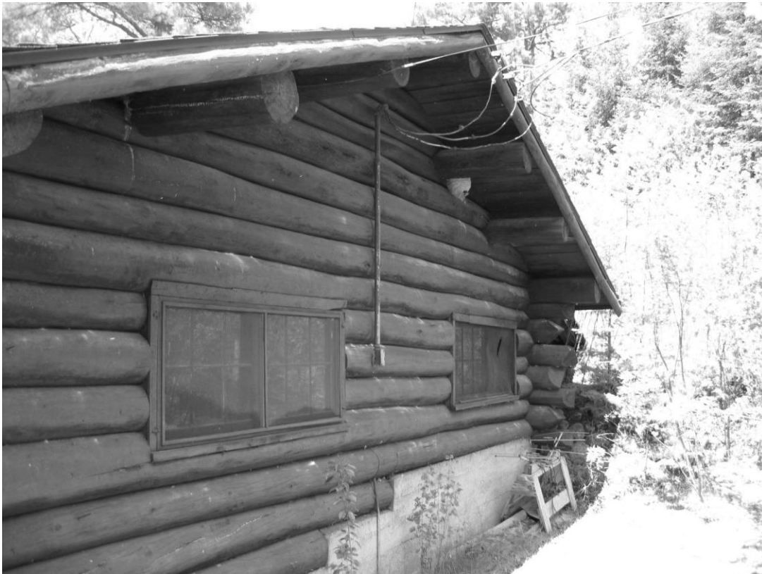
10 of 18. Warehouse (FS Bldg. #31107); Contributing. Eastern elevation. Lake County, MN.
