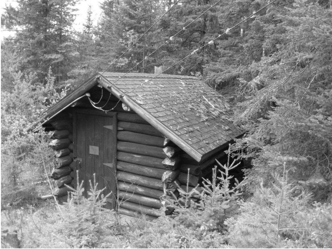
13 of 18. Pumphouse (FS Bldg. #31102); Contributing. Southwestern elevation. Lake County, MN.
