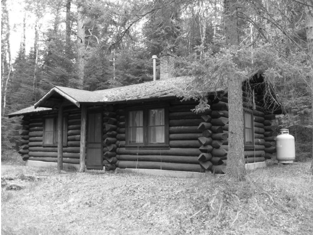
5 of 18. District Office (FS Bldg. #31105); Contributing. Western elevation. Lake County, MN.
