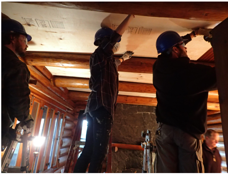
Corpsmembers and staff work on the first step to reinforce the second floor by first adding plywood
