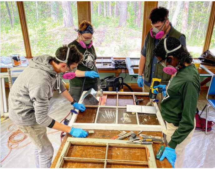
Corpsmembers learning to use a heat gun to remove old glazing
