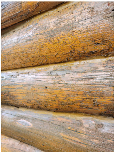
Freshly scraped logs ready for a fresh coat of paint
