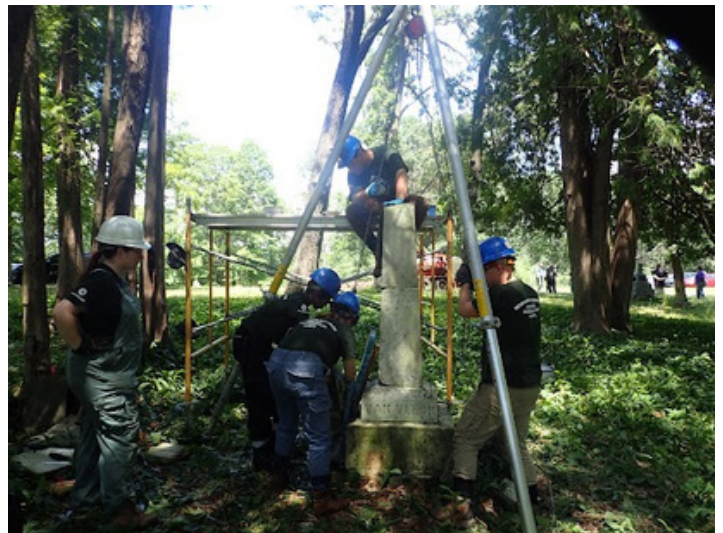
Corpsmembers working to repair a monument using a tripod
