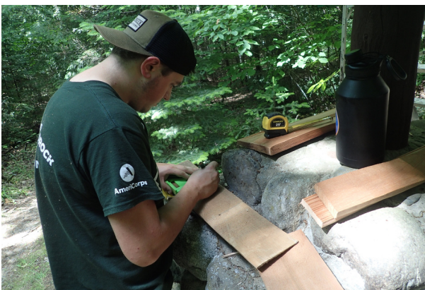
Corpsmember measuring the cut mark on a cedar shake
