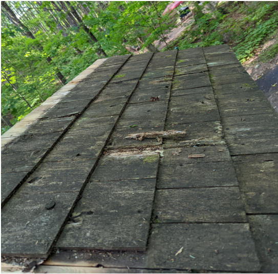
A roof needing new cedar shakes
