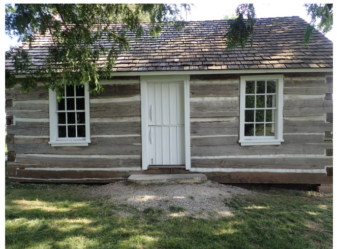
Front view of the cabin with some new mortar
