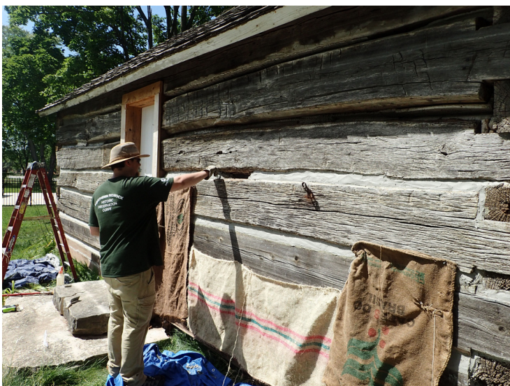
Corpsmember applying new mortar to the cabin
