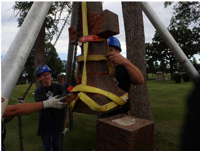
Corpsmembers using a tripod to reset a top piece of a monument
