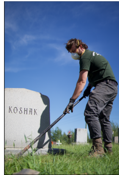
A Corpsmember using a rock bar to reset a monument
