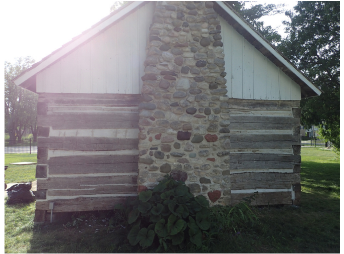
After picture of the chimney side with new mortar
