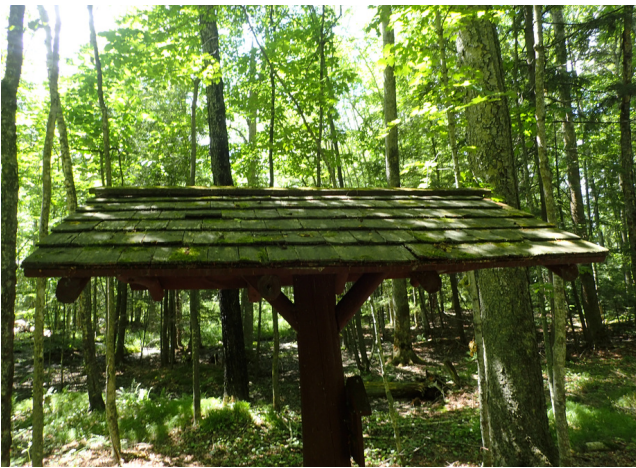
Franklin Lake well roof that needed new cedar shakes.
