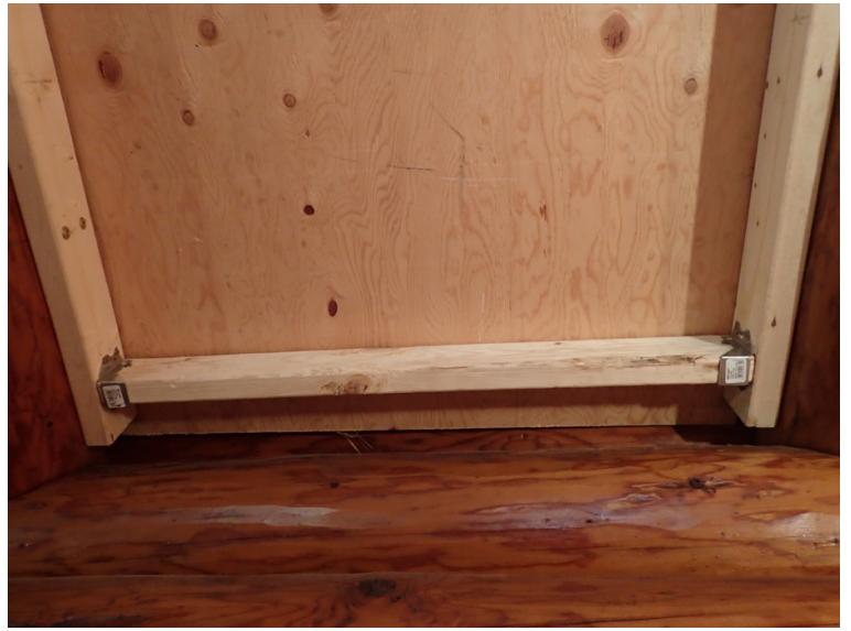
Joists are attached to ledger boards along each log to distribute the load
