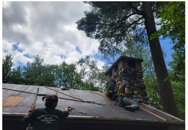
Corpsmembers learning to install rolled roofing
