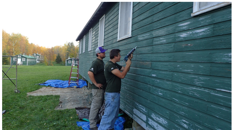
Two Corpsmembers caulking some checks in the wall
