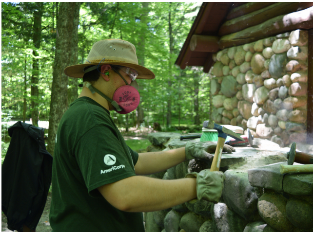
Corpsmember chiseling away old mortar on the comfort station wall
