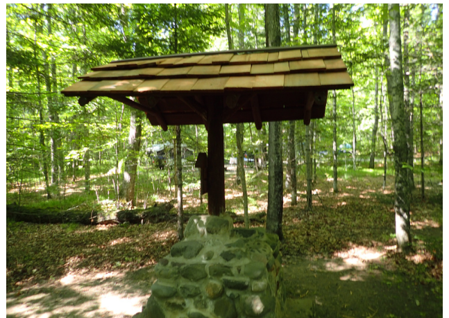
Picture of well roof with new cedar shakes
