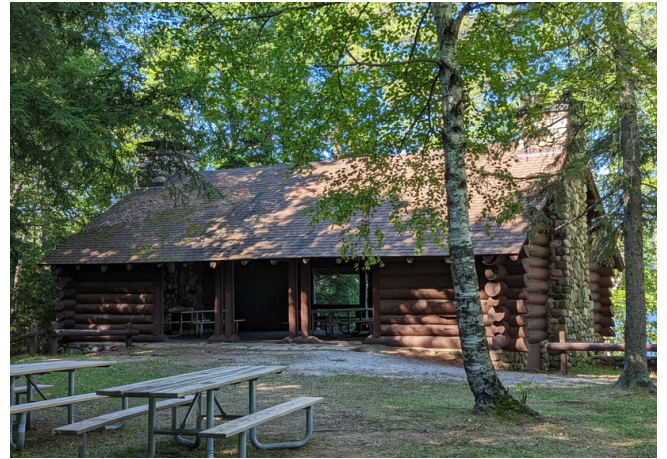
A building needing a borate application and roof cleaning
