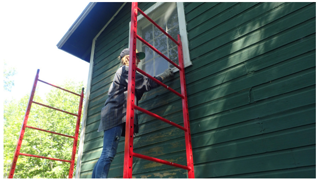
Corpsmember scraping window trim for a new coat of paint
