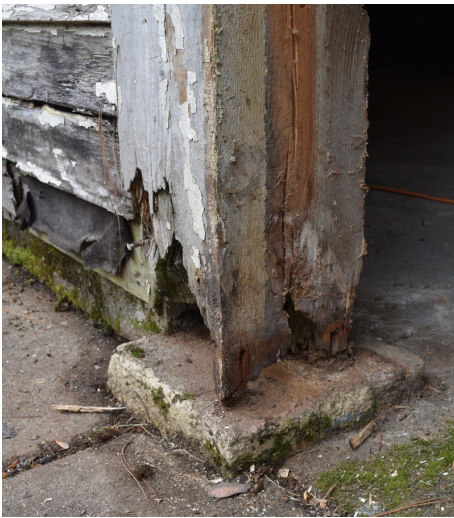
A damaged structural beam for the Corpsmembers to replace
