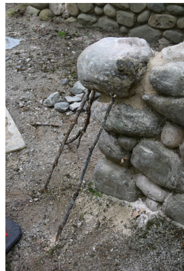
Picture of Corpsmembers' ingenuity using sticks to support a reset stone
