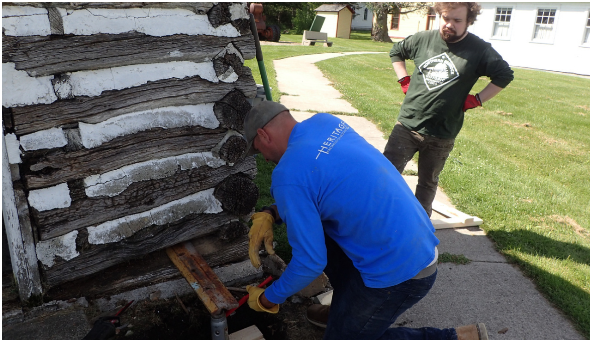
A Corpsmember learning from a Technical Instructor how to use grader blades in log replacement
