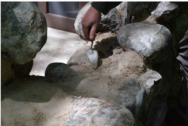
New mortar placed for wall reconstruction
