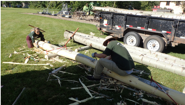
Corpsmembers prepping a log by stripping the bark off
