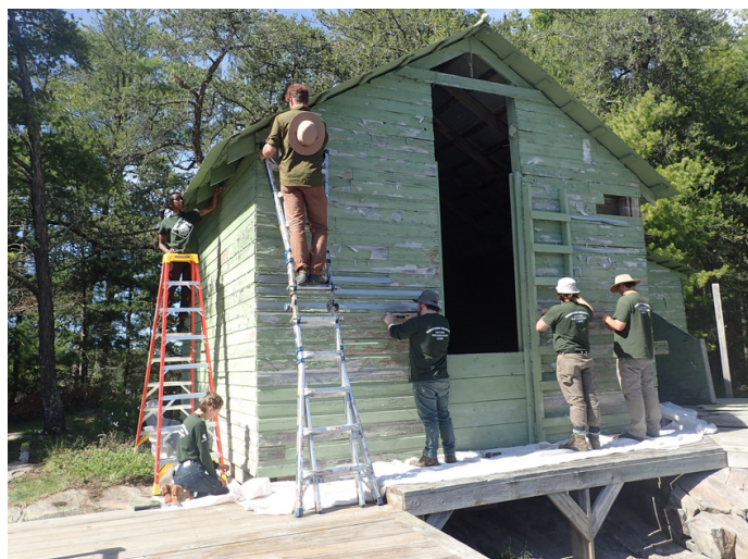
Corpsmembers scraping a building before painting
