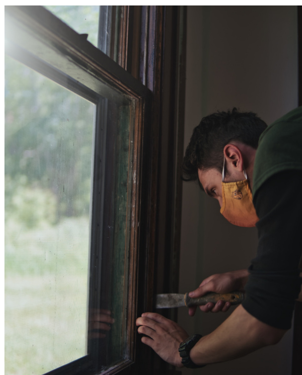
Corpsmembers working to remove wooden sash
