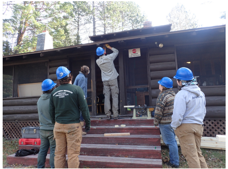
A staff member demonstrates the second step of reinforcement by showing how to measure angles to create wedges that will keep the ledger boards plumb
