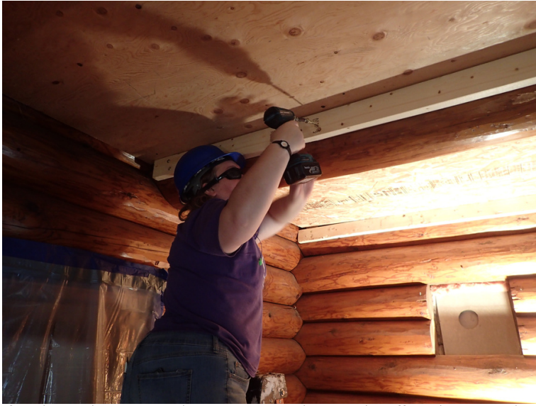
After the wedges are in place, Corpsmembers and staff work on attaching ledger boards to each log
