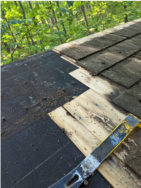
The process of removing old cedar shakes
