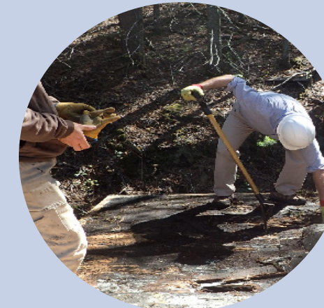
Repairing District Office Roof
