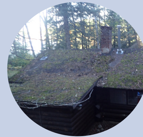
District Office Roof (Before)
