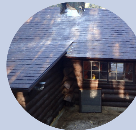
District Office Roof (After)
