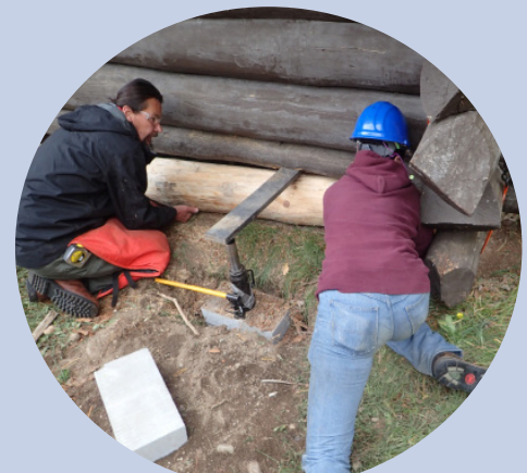
Warehouse Log Replacement
