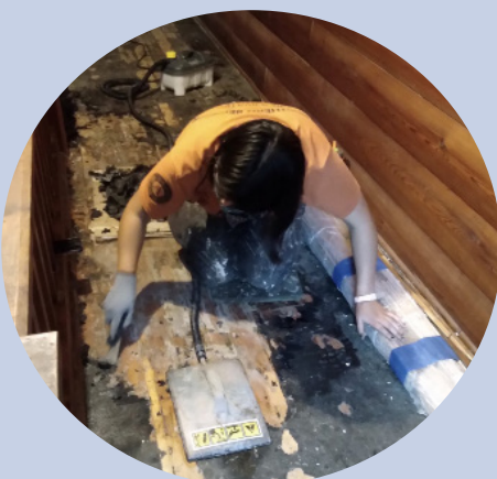
Ranger Dwelling Floor Restoration
