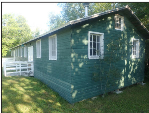
Mess Hall - Before
