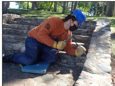
Mortar Removal
