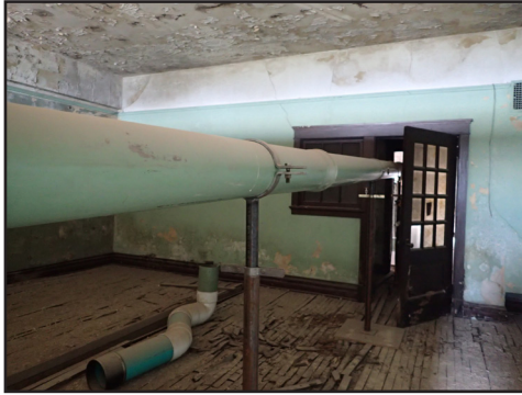
Pipe Removal - Before
