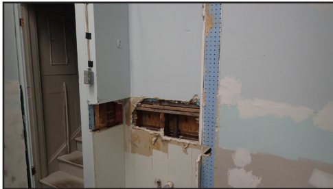
Doorway Demolition - Before
