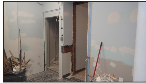
Doorway Demolition - After
