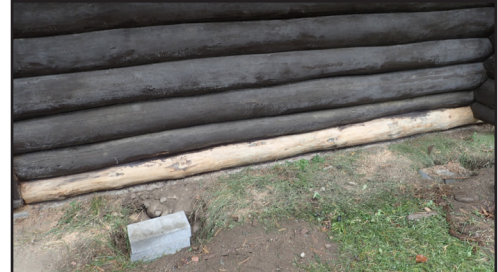
Warehouse Log Replacement After
