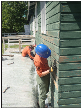
Mess Hall - During
