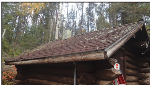
Pump House Roof Before
