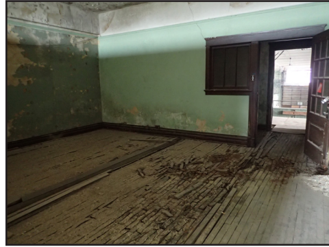
Pipe Removal - After
