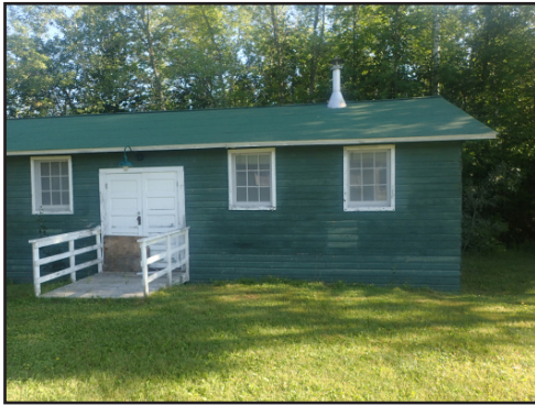
Mess Hall - Before
