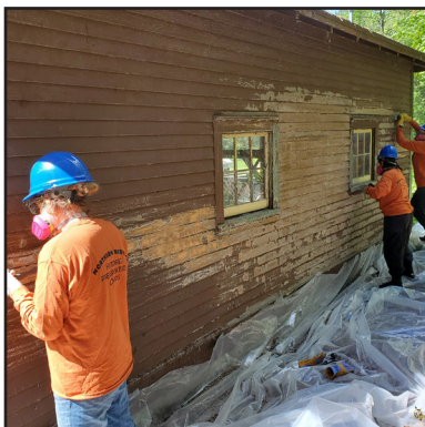
Scraping and Painting
