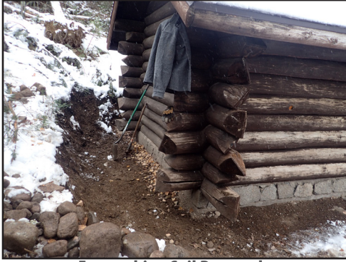
Encroaching Soil Removal
