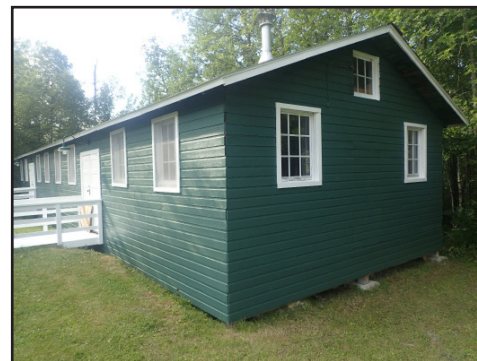
Mess Hall - After
