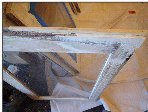
Wood Epoxy Repair
