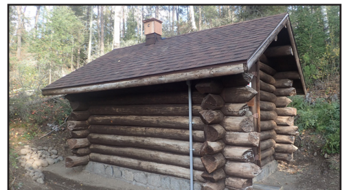
Pump House Roof After
