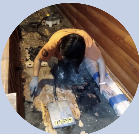
Ranger Dwelling Floor Restoration
