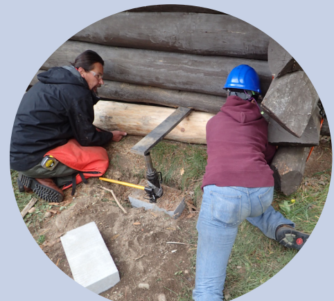
Warehouse Log Replacement
